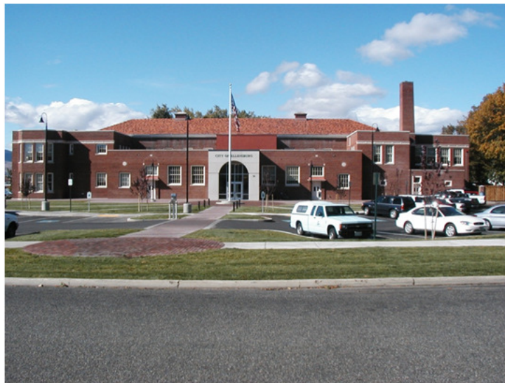
The New City Hall. The City completed the renovation of the old Washington Elementary School in 2005. In staying true to our past, the City renovated the building to meet the City’s needs without having to tear the building down. The exterior remains intact and on the national historical register.
